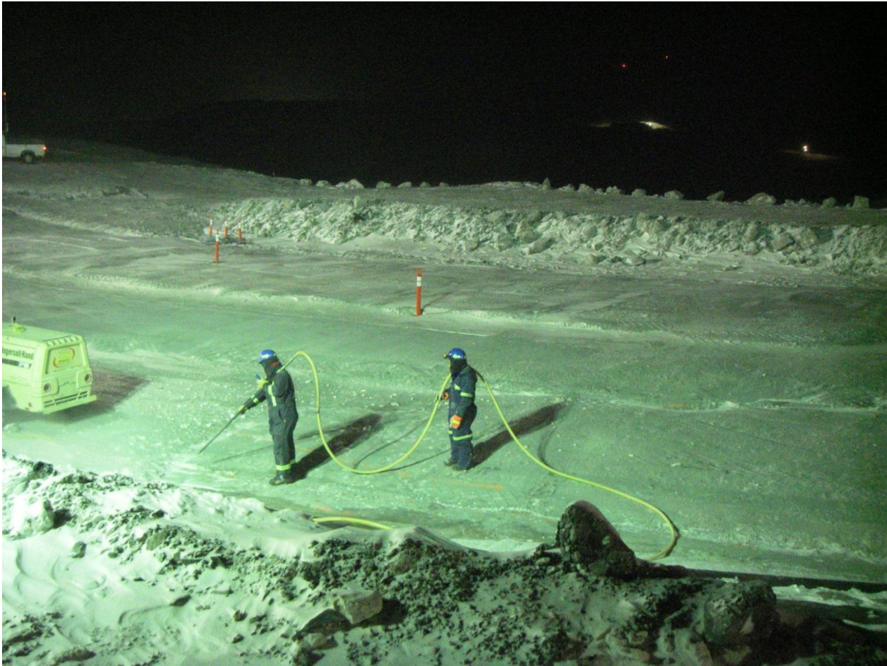
Photo 6: Laborers cleaning snow and loose gravel using compressed air.
