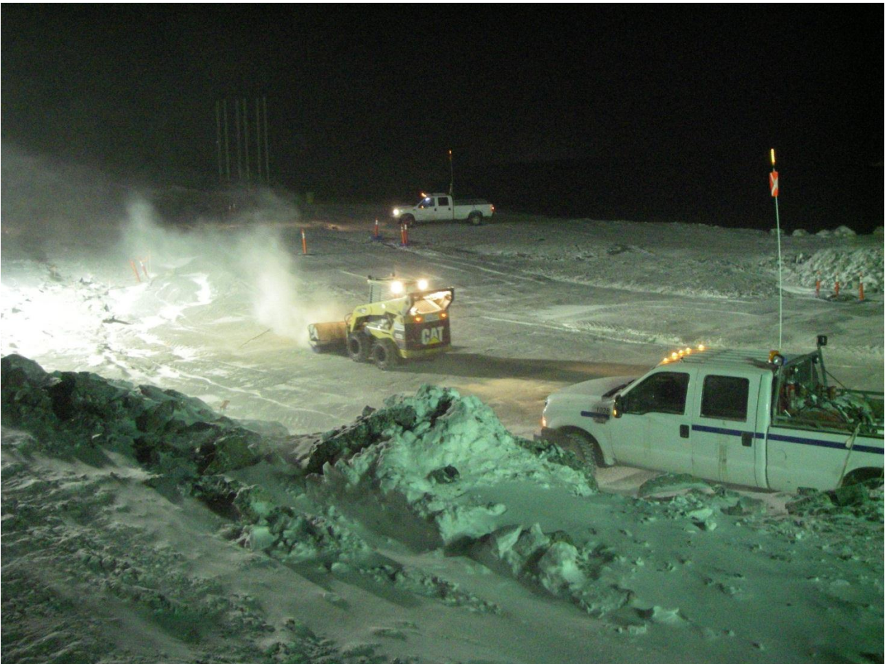
Photo 7: Skidsteer equipped with broom attachment cleaning loose gravel and snow from frozen core area.
