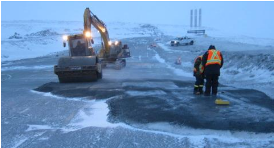
Photo 4: Trial placement near the center of the key-trench.
